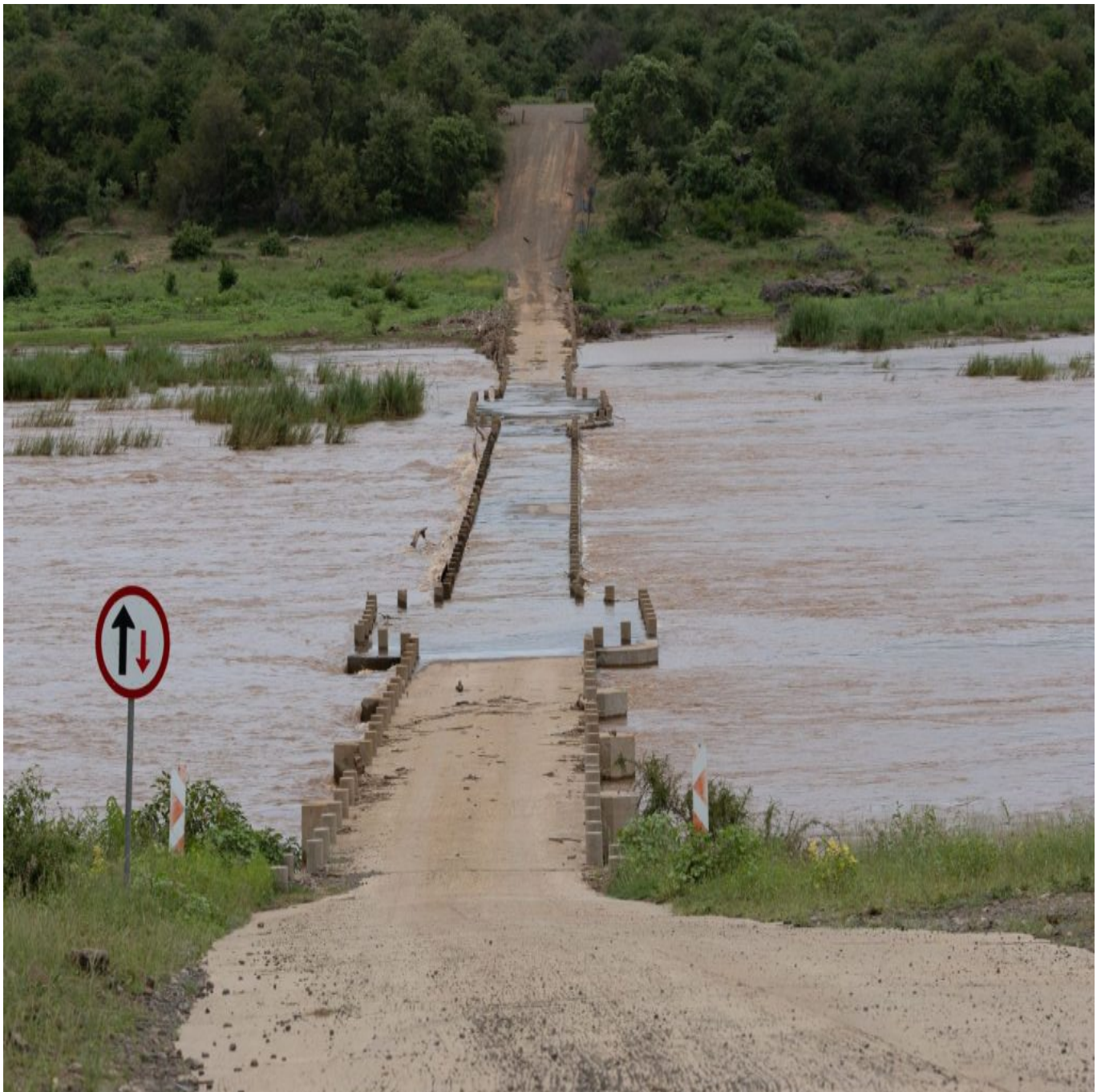
Balule low-water bridge overstroomt
