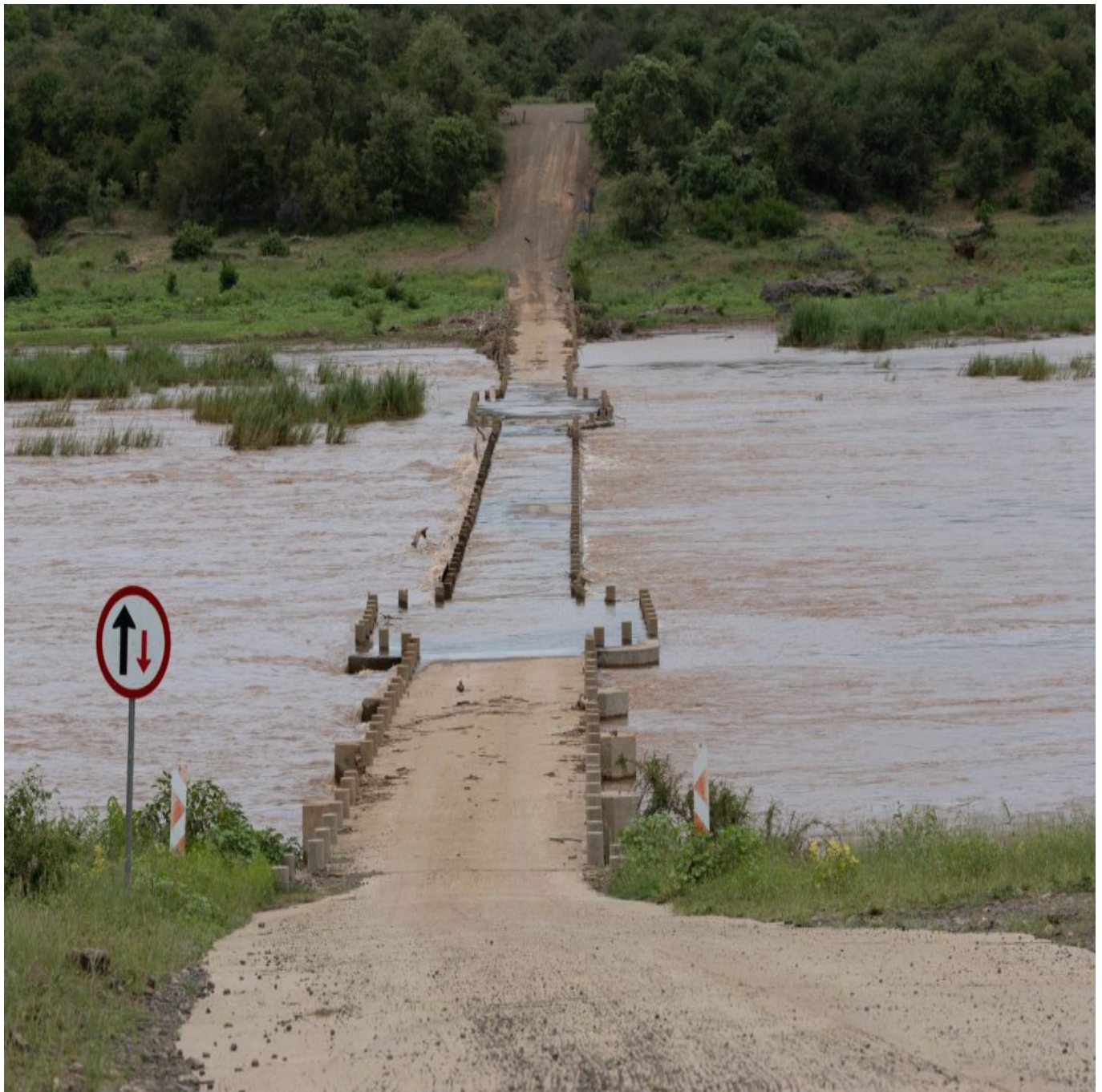
Balule low-water bridge overstroomt
